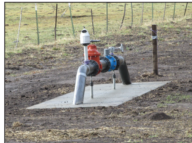
Above: The newly piped water delivery system. Before, irrigation water was distributed via an open ditch. Below: The new water intake for the irrigation system, which serves four landowners. (Photos: USWCD)
