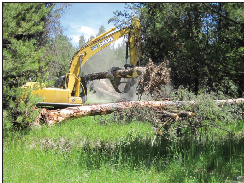
Above: Trees with rootwads are used for large wood structures, providing valuable habitat for salmonids. (Photo: USFS)
